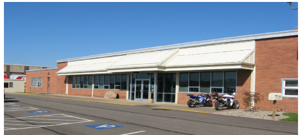
County Engineers Windows/ Doors Replacement
