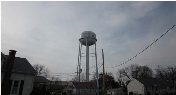
Village of Beach City Water Tank
