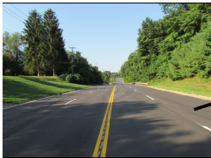
Everhard Rd. Repaving
