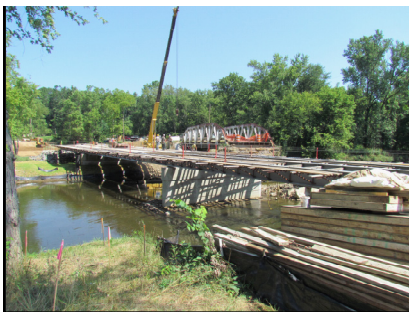
Riverland Ave. Bridge Replacement
