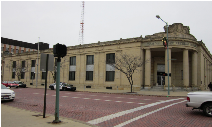
Historic Building - Frank T. Bow Federal Building
