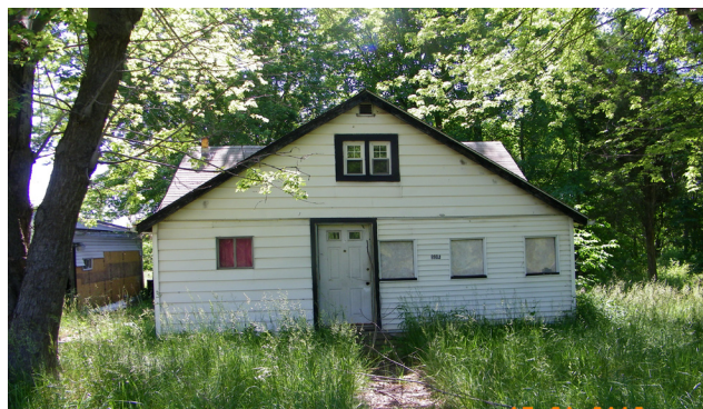
Bethlehem Township Demolition
