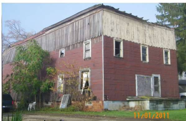
Village of Beach City Demolition
