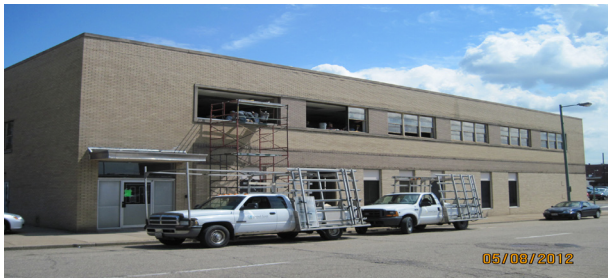
Data Center Window Replacement
